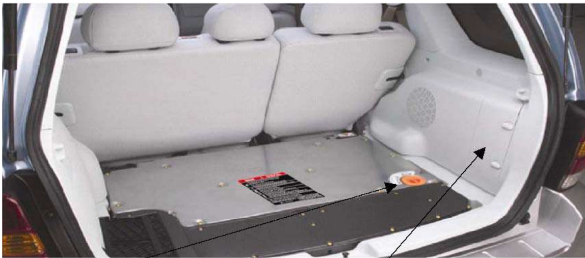
High voltage Service Disconnect Switch
