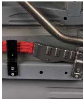
Thermal shield near hot exhaust
