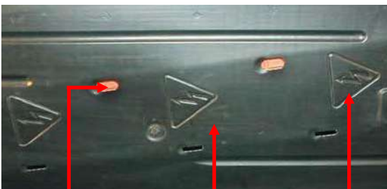
High-Voltage Cable Visible
