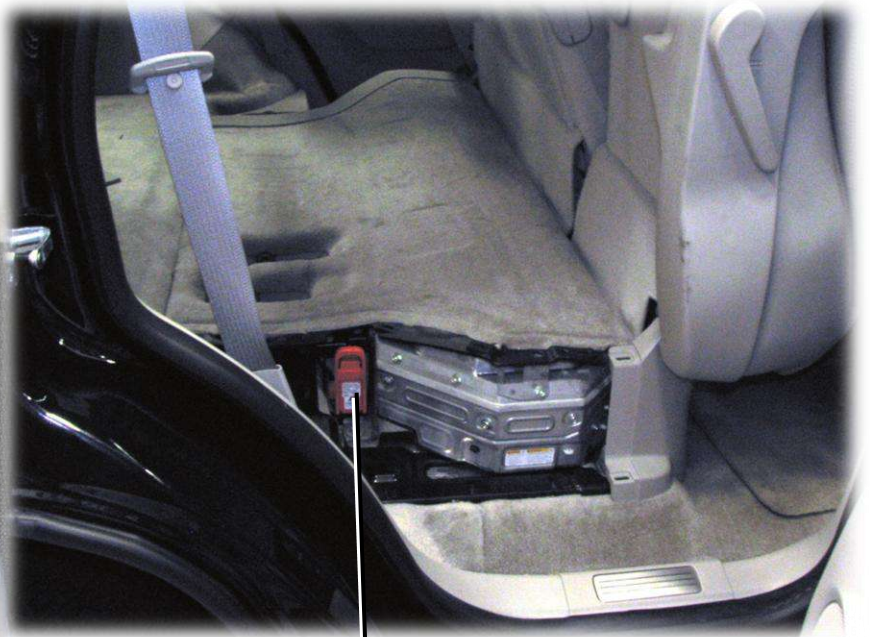
300V Hybrid Battery Manual Disconnect
