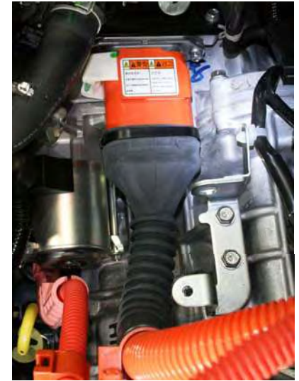
High-Voltage Cable Connection to Motor
